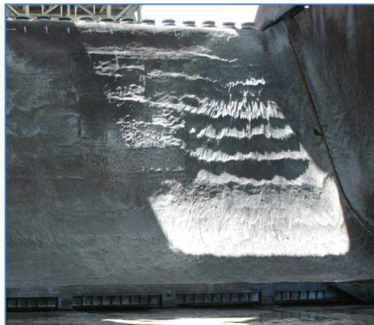
Fig. 32 Scallop created by the SRB plume on the refractory concrete before the STS-133 refurbishment.
